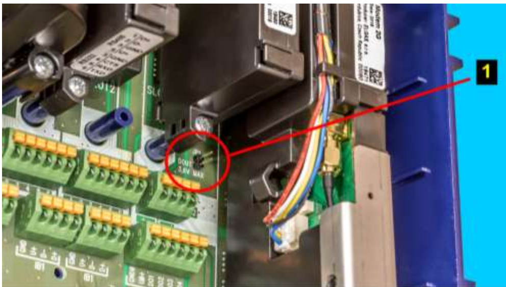
Fig. 41: Placing JP1 Jumper on I/O Board
