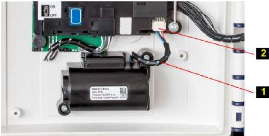
Fig. 25: Connecting the device battery
