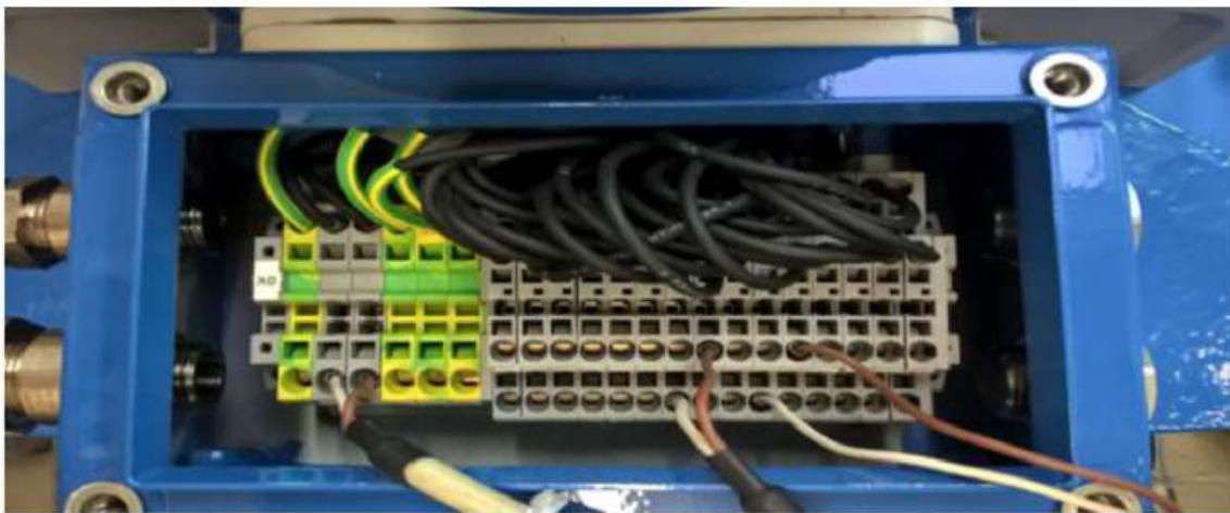
Fig. 8.19: Connection of the RS 485-2 (22 +, 23 -) at the USM GT400
