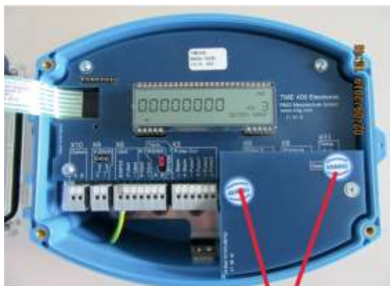
In the electronic enclosure
