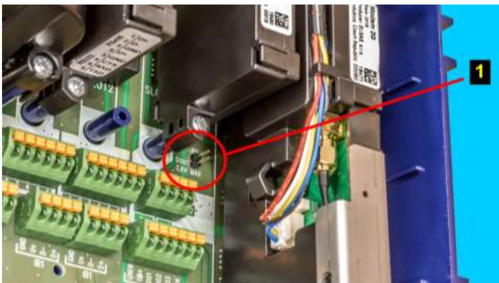
Fig. 41: Placing JP1 Jumper on I/O Board
